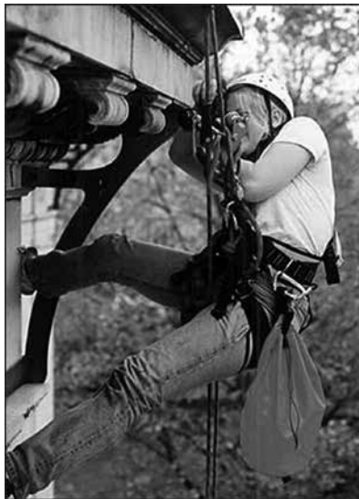
Susan Knack, a civil engineer for Simpson Gumpertz & Heger, rappels down buildings to examine its construction for various problems or conditions.
