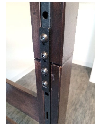
Figure 5 Connecting Plate with Frame Bolts
